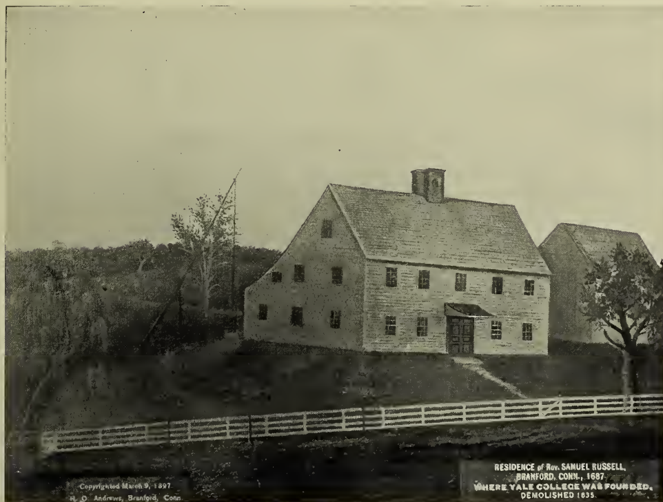
OLD HOUSE IN BRANFORD
